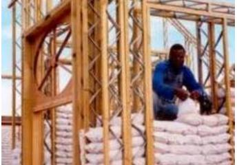
Fig. 3.9: The Eco-Beam and sandbag system by engineer Mike Tremeer (earthbagbuilding.com/articles/eco-beam.htm)
