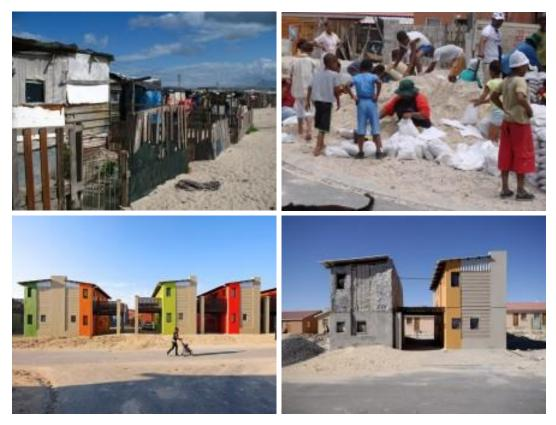
Fig. 3.10: The 10×10 Sandbag Houses by architect Luyanda Mpahlwa & others (designother90.org/solution/10x10-sandbag-house/)
